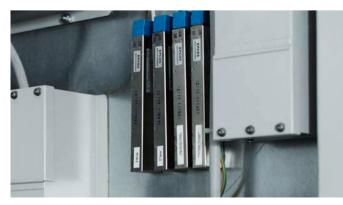
filtered, it is suitable to install the single filters into boxes (up to maximum 52 pairs of lines) or into cabinets (up to maximum 500 pairs of lines). This preparation will simplify future filter upgrades and allow entry to the shielded area with multi-core cabling.
