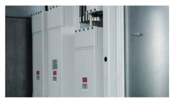
The high capacitances between the lines and ground require special protective measures. If there are no product-specific requirements, protection with a secondary ground wire (cross section min. 10 mm<sup>2</sup>) in accordance with EN 50178, is necessary. For this purpose, the filter case has connecting bolts at each end. Resistors are incorporated in the filter to discharge capacitors after shut-down.
